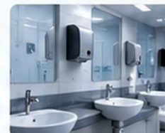
RESTROOMS Fixtures, handles & surfaces
